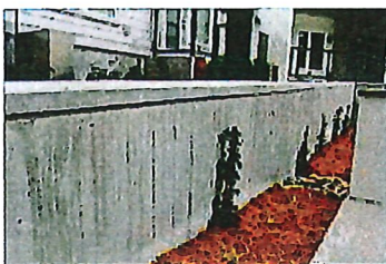
board form concrete walls
