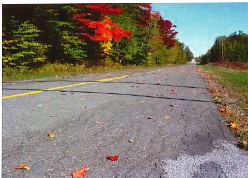
Traffic Counts Burgess Road, Hayes Township
